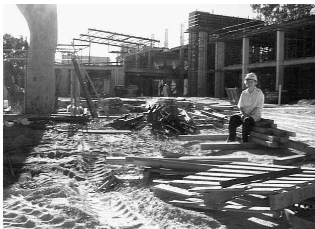
Anne Batt, Medical Librarian, on site at the new Medical Library. Architects: Hames Sharley. Builders: BGC
