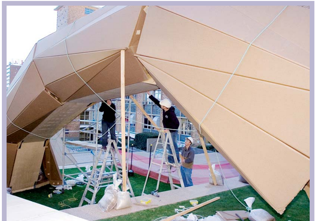
Students work on the tri-wall multicell cardboard cladding supplied by Visy Board.
